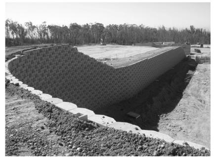
*Figure 16.1* Example segmental block wall
