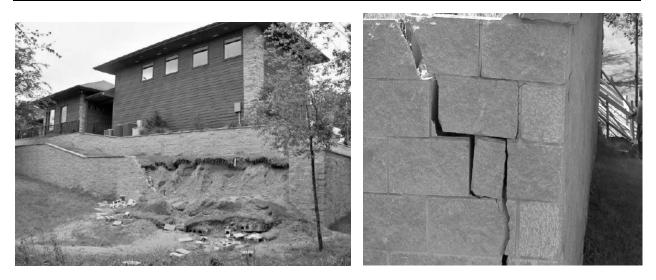
The above photo is a rare occurrence. No building permit, not engineered, minimal reinforcing in ungrouted cells, and other oversights.
