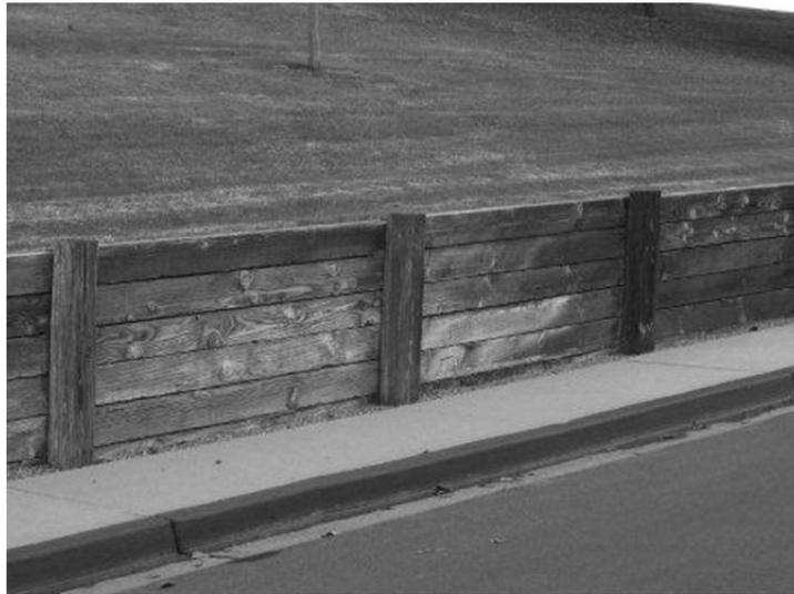
*Figure 13.1* Typical wood retaining wall
